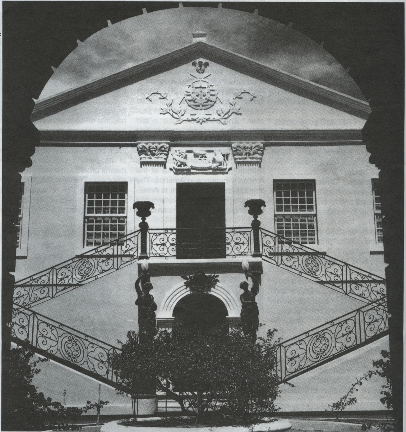
A fine example of eighteenth-century Portuguese architecture on Mozambique Island
